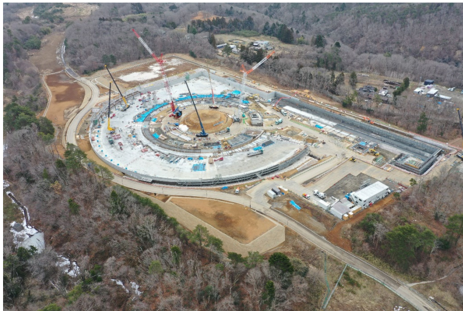
Figure 1.4 Aerial picture of the construction site of the NGSR facility as of 28-Jan-2021 (by courtesy of PhoSIC).
